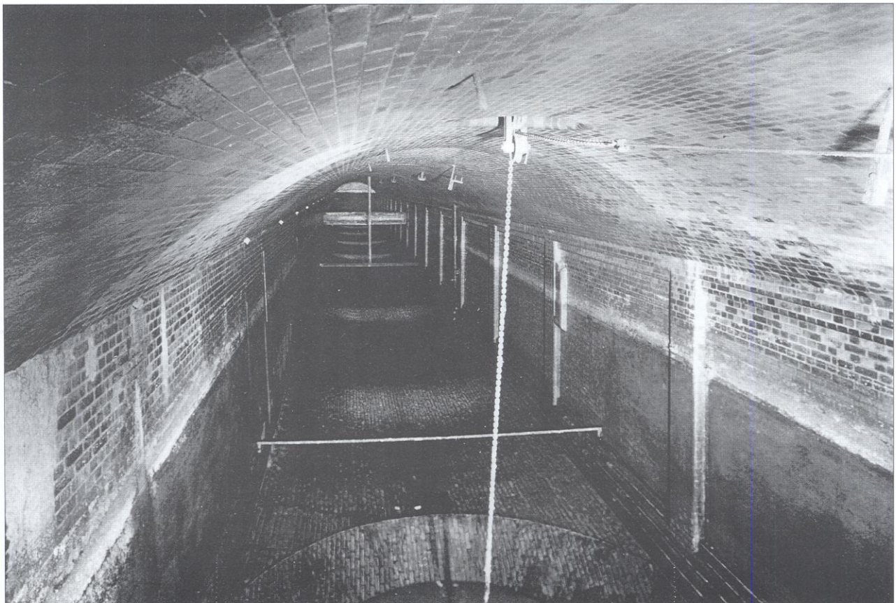
One of ten underground sedimentation tanks, with a capacity of 1,200 cubic metres.
