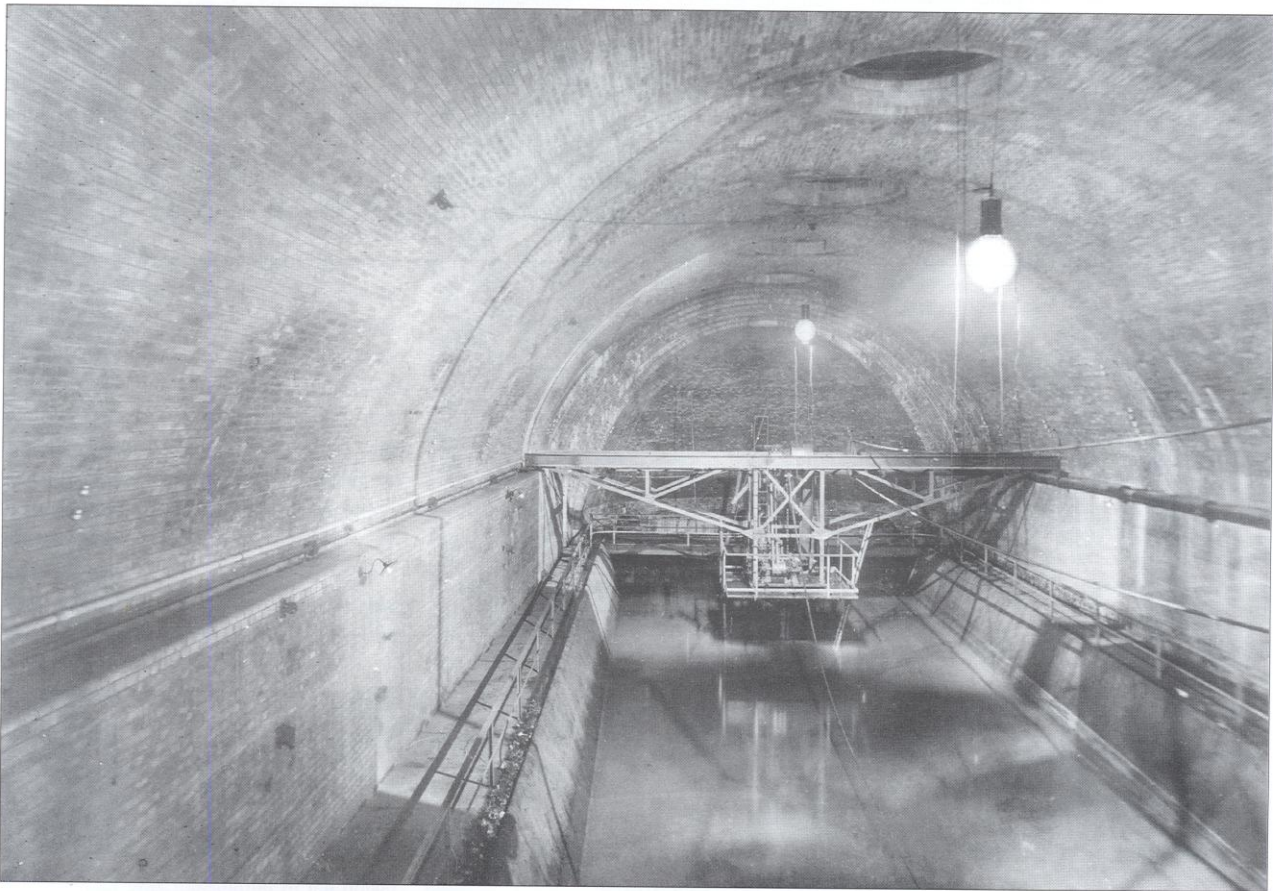
The sand trap hall during a trial run in 1906. The screens along its edge can be seen, as well as piles of screenings in the grooves.
