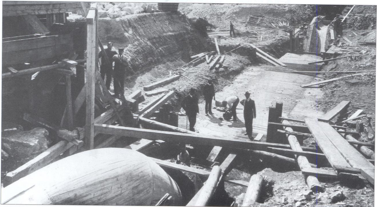
Construction of a smaller inverted siphon in Prague.
